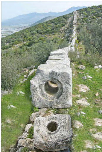
Figure 1.2: Photograph of a stone pipe of Patara's aqueduct, in Turkey [87].
